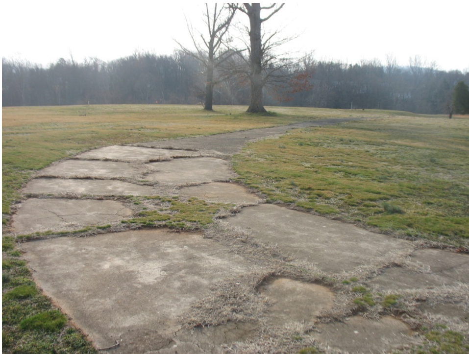
Field Photo 41: Concrete Path. View looking east.
