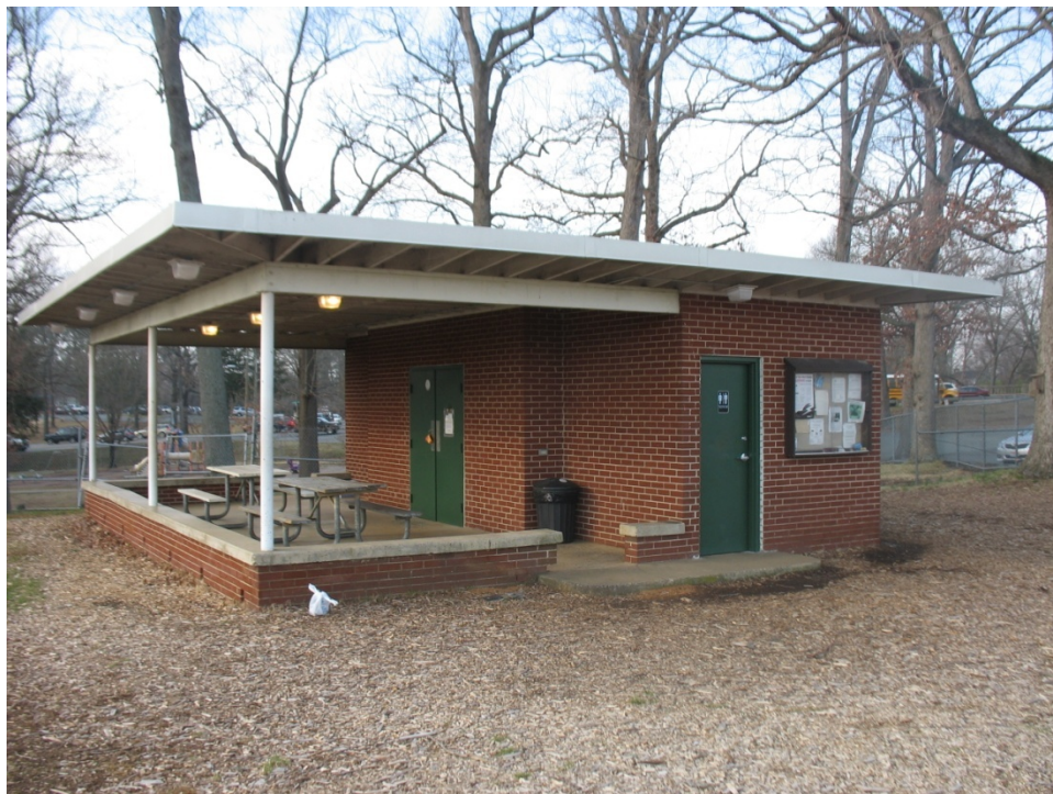
Field Photo 49: Club House. View looking south.
