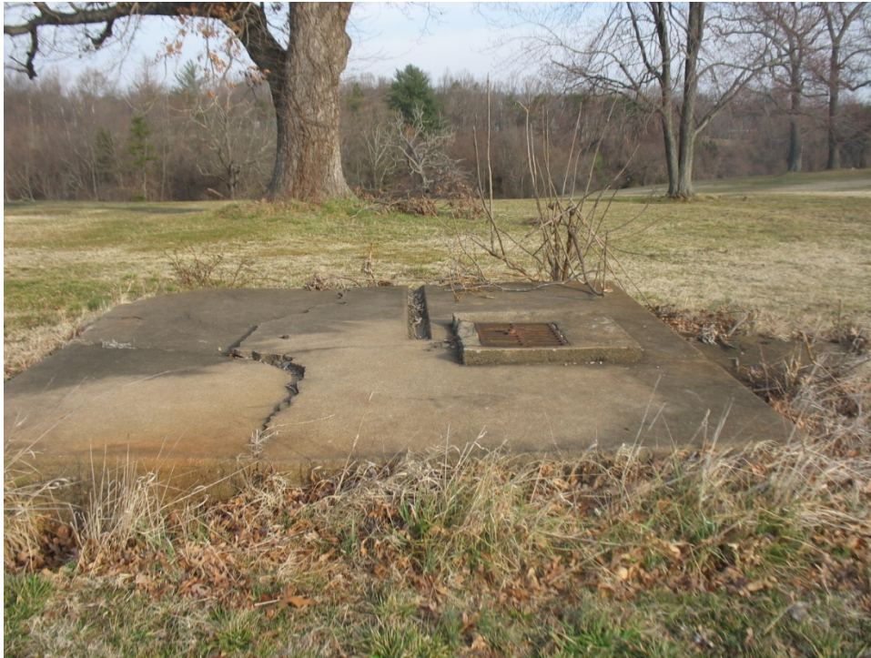
Field Photo 47: Concrete Foundation. View looking west.
