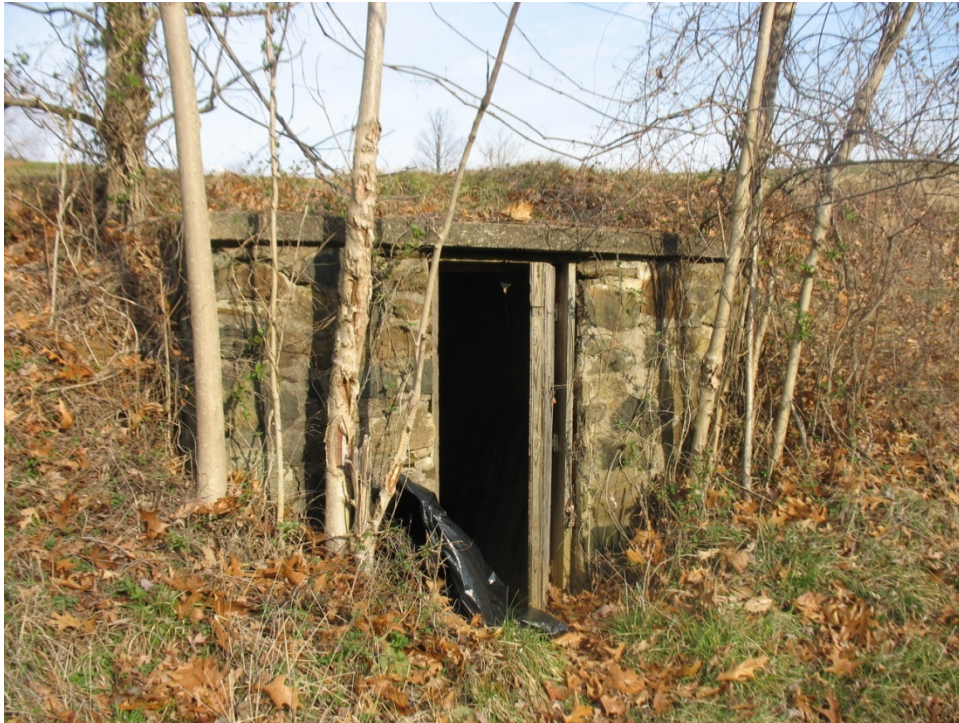
Field Photo 50: Stone Building. View looking west.
