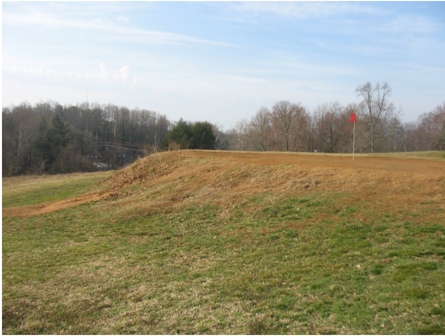
Field Photo 4: First Green Terrace Wall. View looking south.
