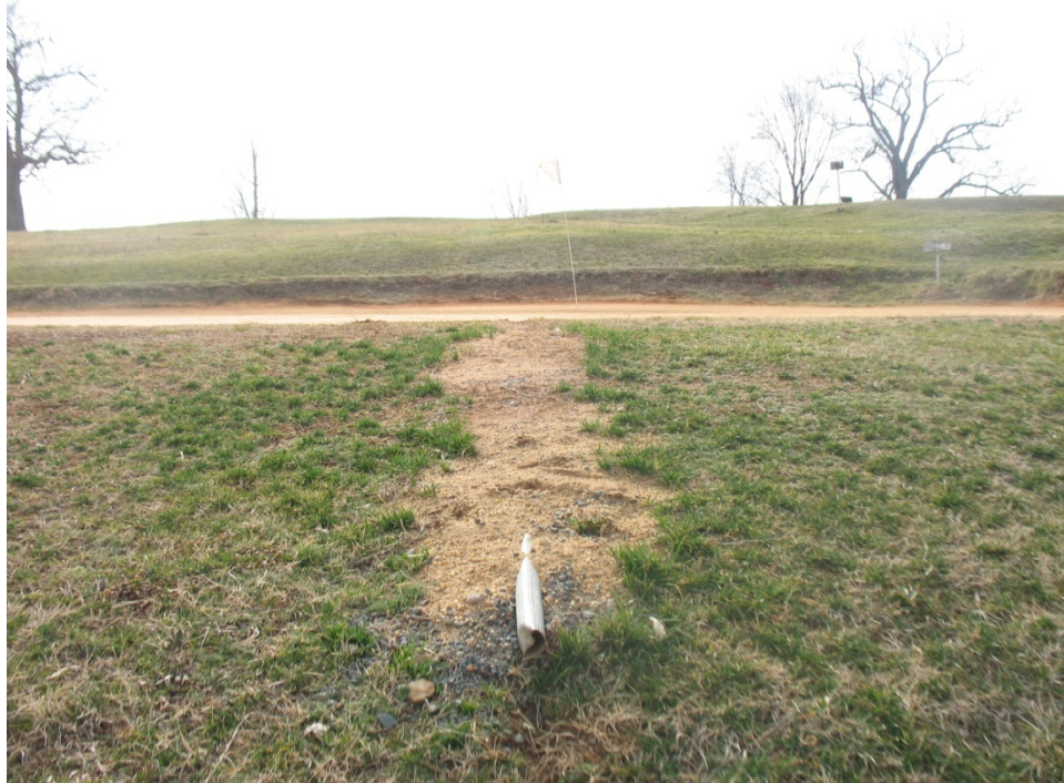
Field Photo 48: Eighth Green Drain Pipe. View looking east.
