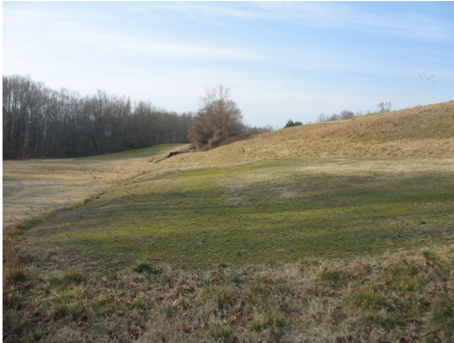
Field Photo 10: Third Hole Landing Area on Abandoned Railroad. View looking south.
