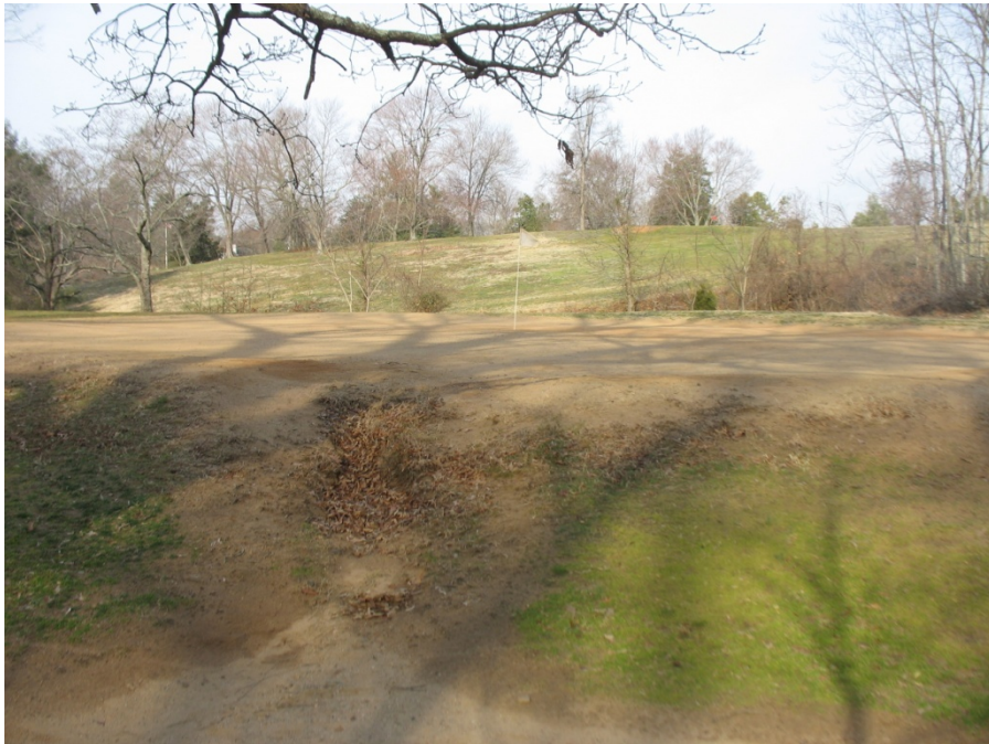
Field Photo 15: Erosion on Fourth Green. View looking west.
