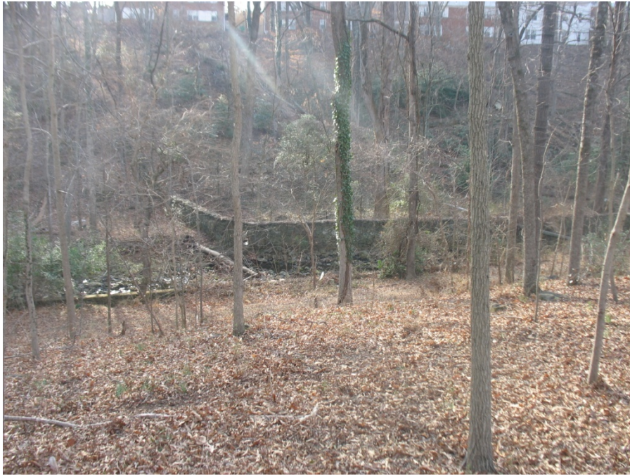
Field Photo 16: Stone Wall at Former Rock Hill Estate. View looking east.
