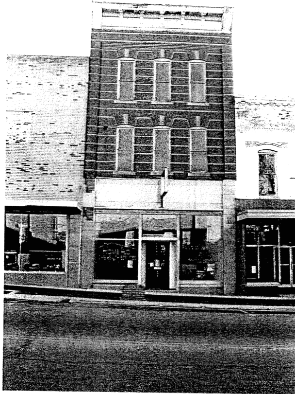
FIGURE 16: Commercial Building, 207 N. Main St. (251-5001-0113)
