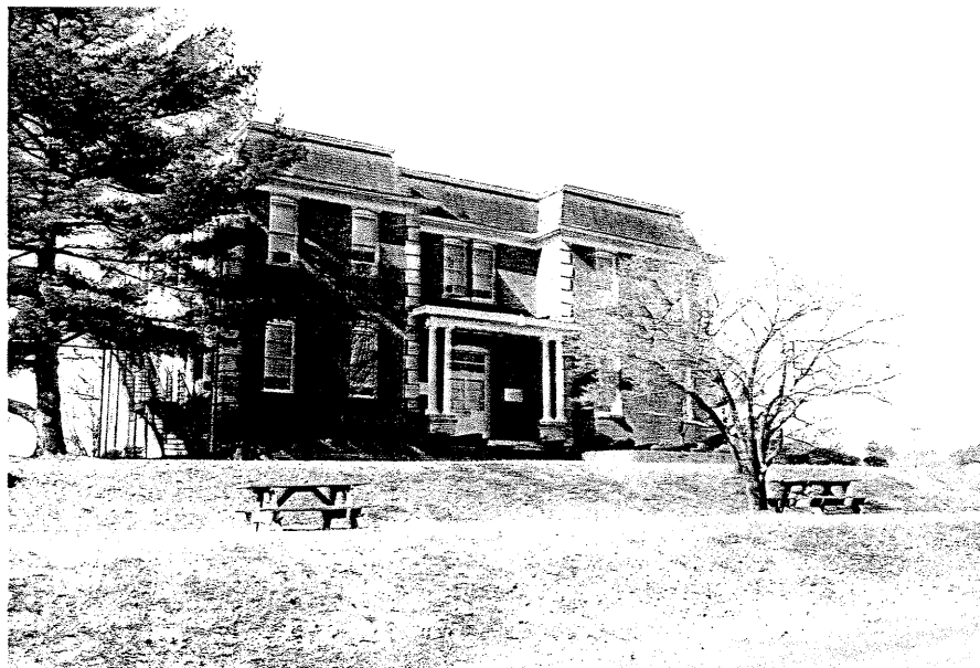
FIGURE 24: Lawrenceville High School, 405 Park St. (251-5001-0214)
