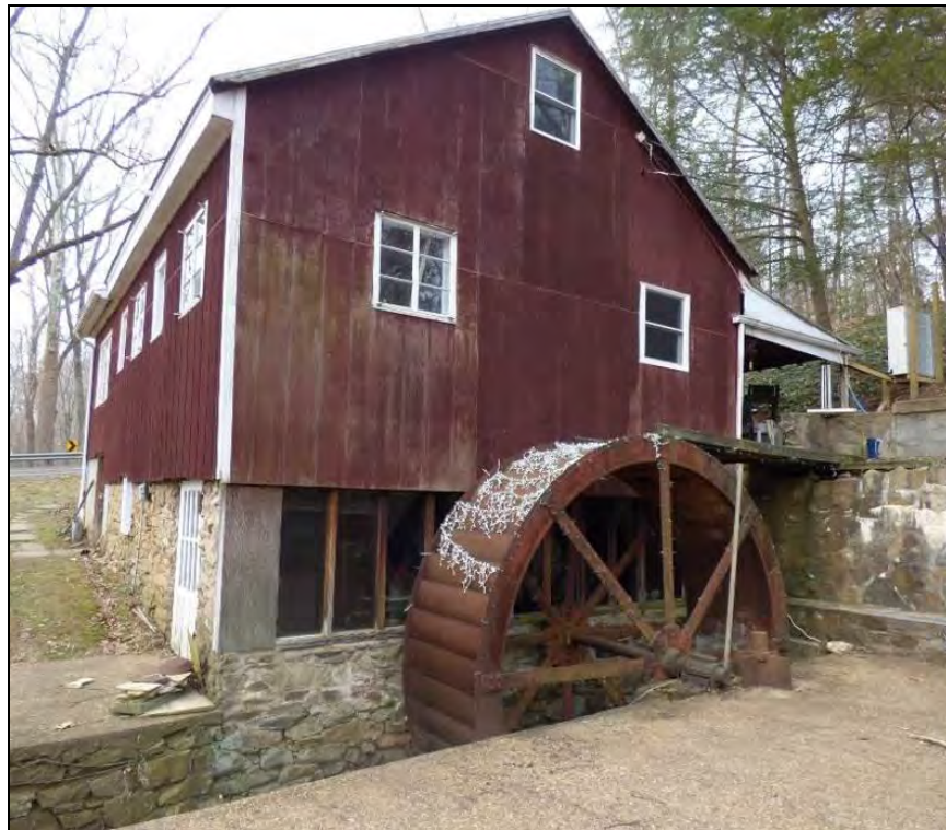
Photo 11: Northeast Oblique of Thompsons Mill (030-0885).
