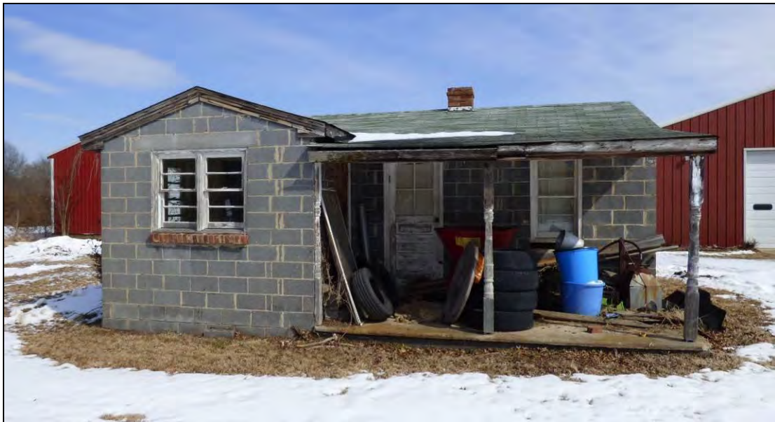
Photo 5: Northwest Elevation of Secondary Dwelling, Robinson House (030-5634).
