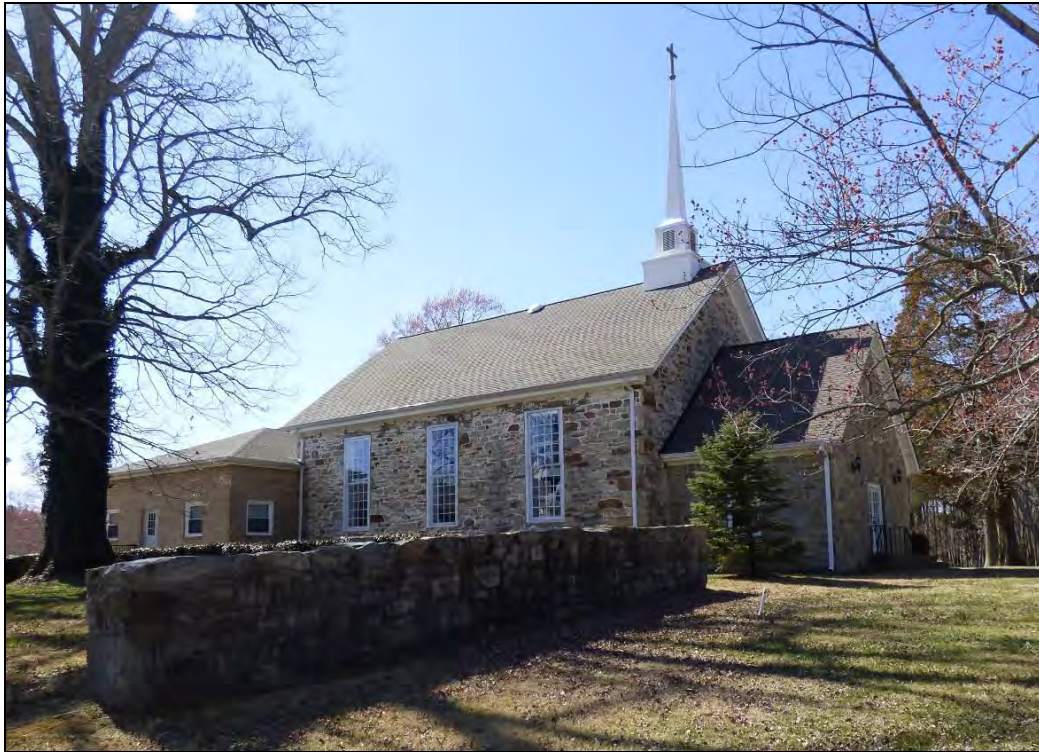
Photo 17: Northeast Oblique of Grove Baptist Church (030-0090).
