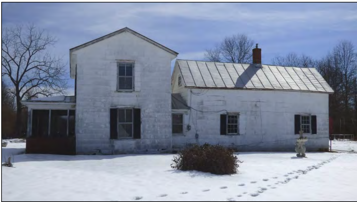
Photo 1: West Elevation of Farmhouse at 11311 Blackwelltown Road (030-5540).
