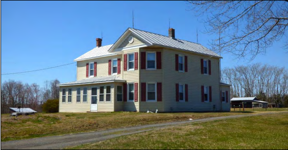
Photo 15: of Marion Cox House at 12960 Blackwells Mill Road (030-5684).
