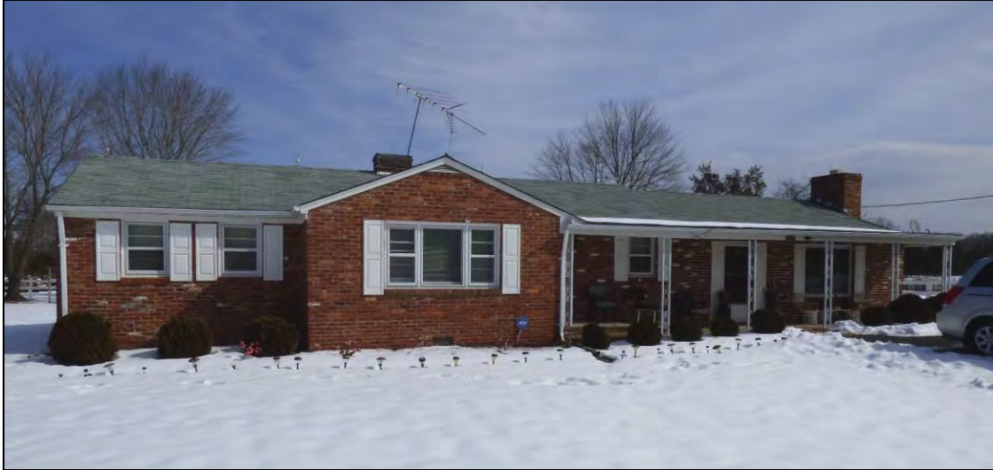
Photo 4: Northwest Elevation of Robinson House at 11207 Blackwelltown Road (030-5634).
