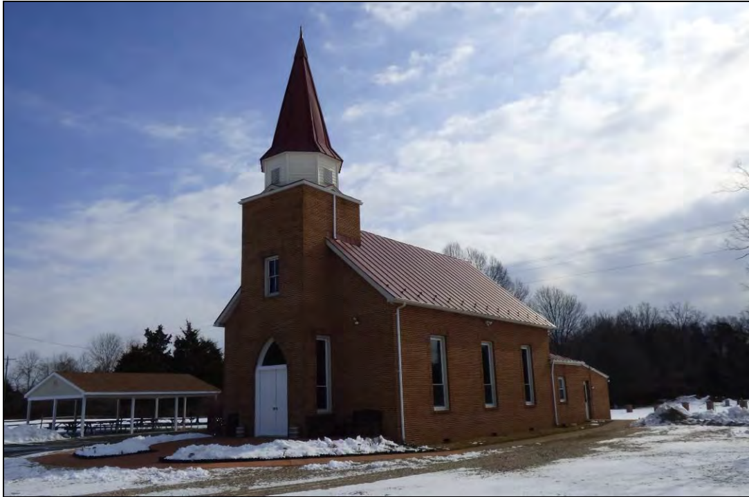
Photo 9: West Oblique of Ebenezer Baptist Church (030-0969).
