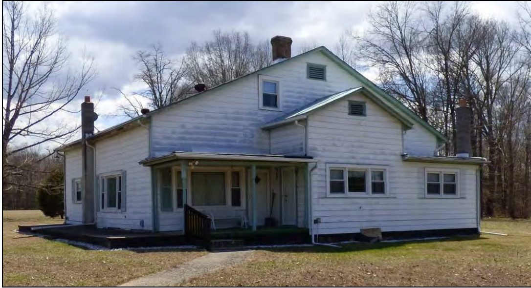
Photo 7: Northwest Oblique, Blackwelltown School/ House at 11363 Blackwelltown Road (030-5541).
