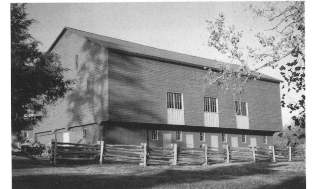
The Bank Barn at Buffalo Springs Farm, after completion of rehabilitation.
