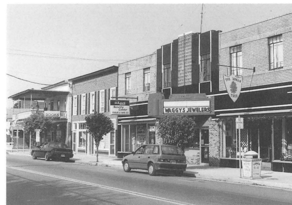
The Mount Jackson Theatre Building is an important landmark for the Shenandoah County town.
