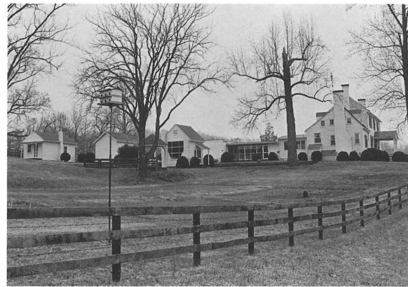
Greenwood is among the earliest I houses built in Orange County. The 19th-century frame dwelling retains its integrity of plan and design.
