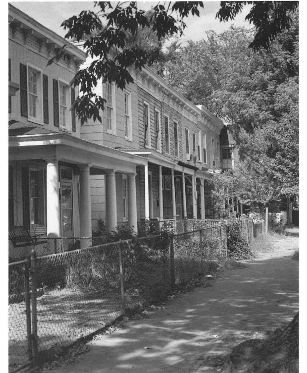
512 South Laurel Street, Oregon Hill Historic District, Richmond
