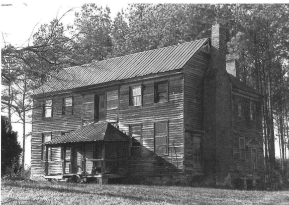
The two-story Bowling-Eldridge House in Halifax County features sophisticated federal styling such as the remnants of a two-tiered pedimented portico.
