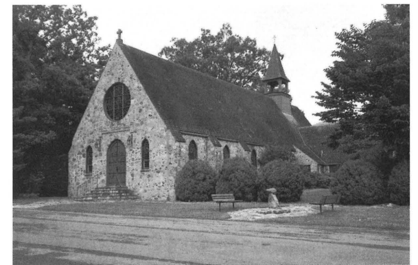
The Chapel at the Blue Ridge School, designed by Ralph Adams Cram, is built entirely of uncut and uncoursed native field stone.
