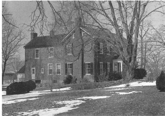
Level Loop, Rockbridge County
