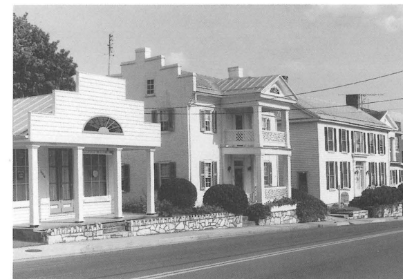
The Tisinger and Pennybacker houses stand on Main Street in the Mount Jackson Historic District in Shenandoah County.
