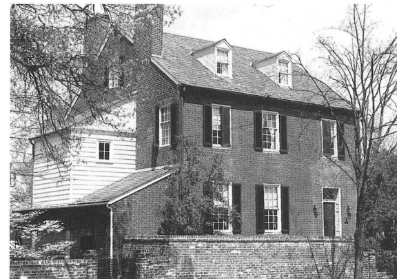
The early 19th-century Dogget House exemplifies the sophisticated town house favored by many of Fredericksburg's professionals.
