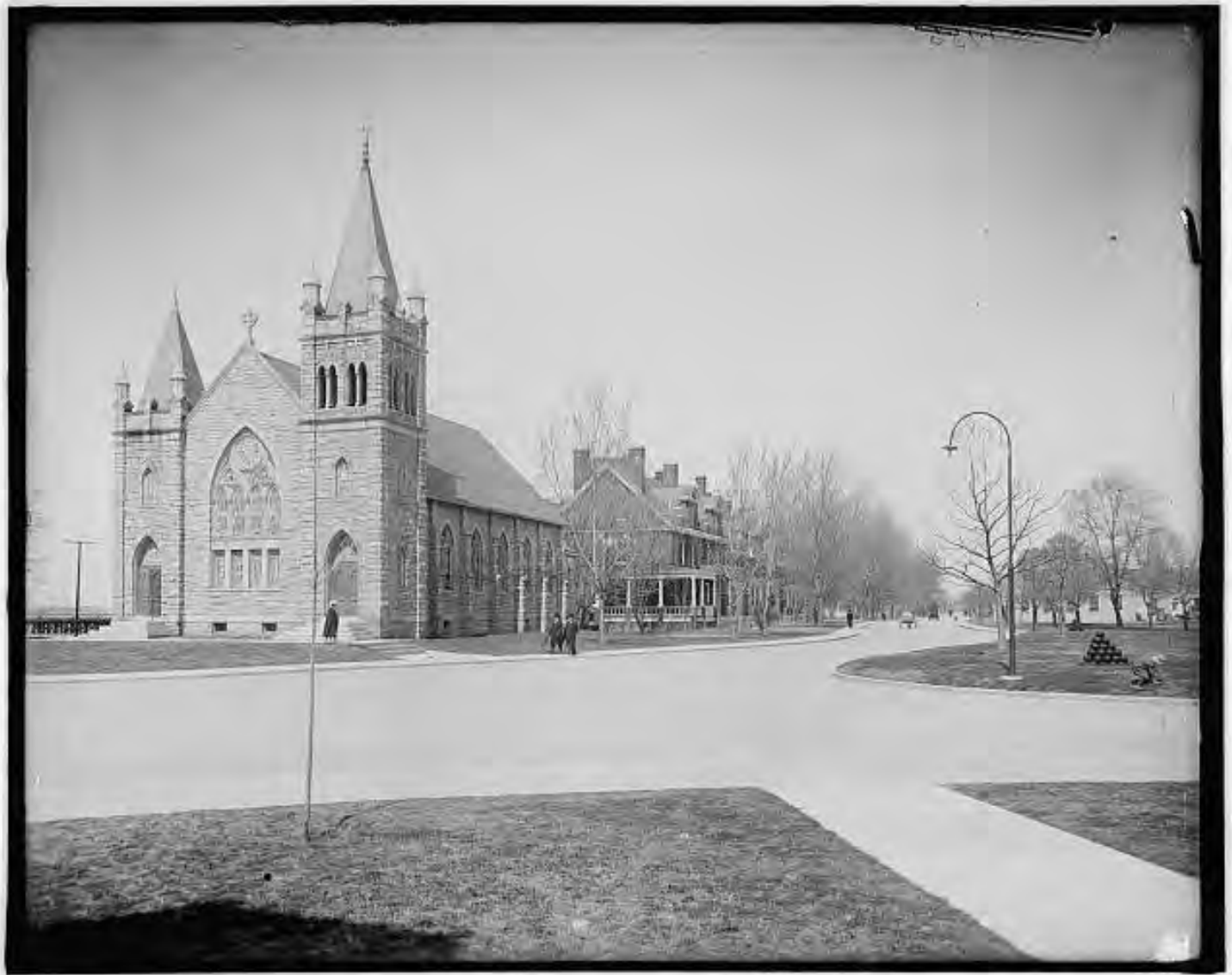
Figure 30. Detroit Publishing Co., Post chapel and officers' quarters, Fort Monroe, Virginia , ca. 1900-1920. Photograph on file with the Library of Congress, Prints and Photographs Division, Washington, DC, https://www.loc.gov/item/2016815777/ .
