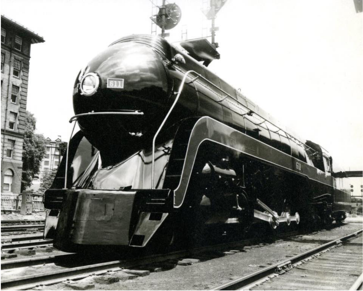
Photo 1: May 29, 1950. The 611 delivery builders photo. Photo: Norfolk & Western Railway
