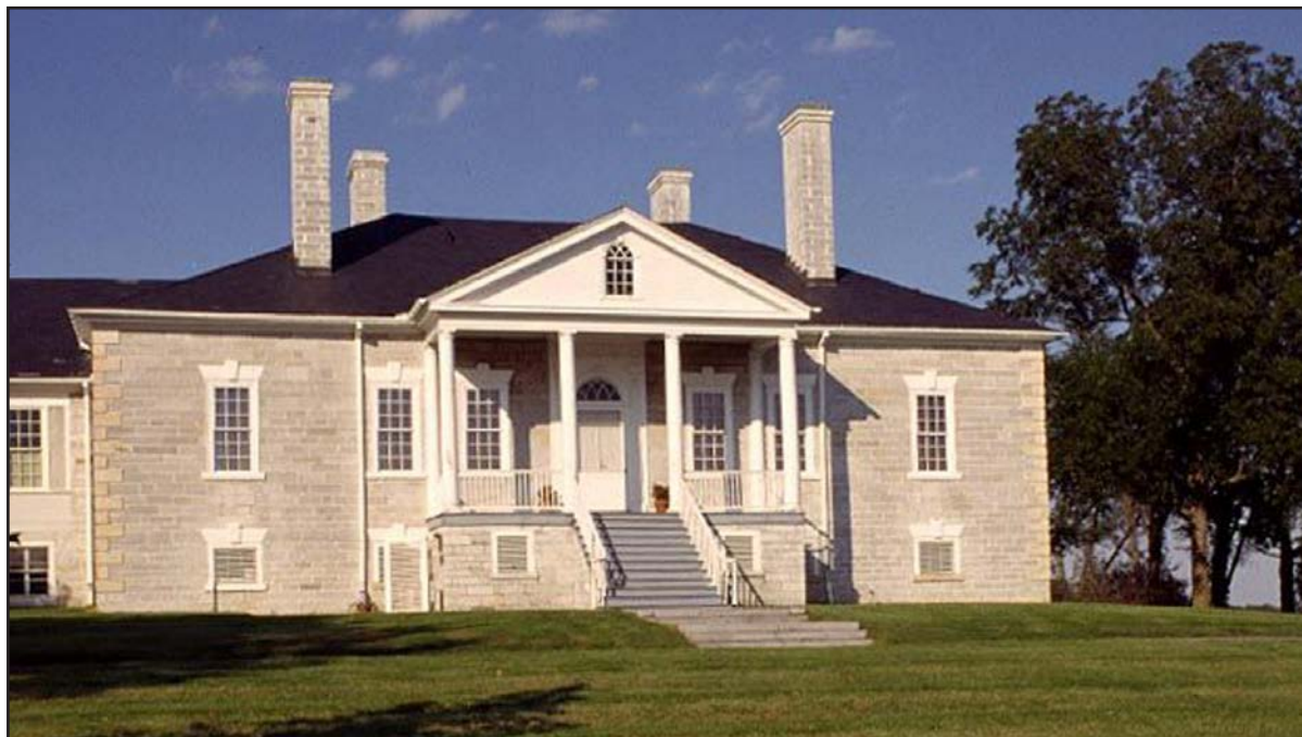
Figure 59. Belle Grove (034-0002), mansion house facade in 2007 (V-CRIS).
