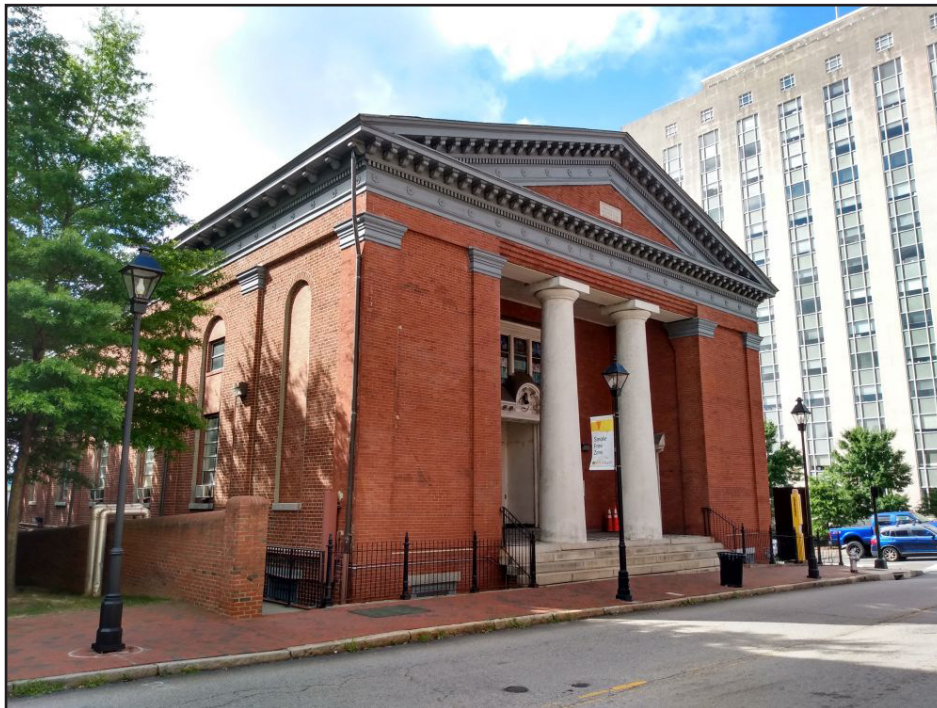
Figure 138. Old First African Baptist Church (127-0167/127-0252), built in 1876 on the site of the 1802 church (V-CRIS).
