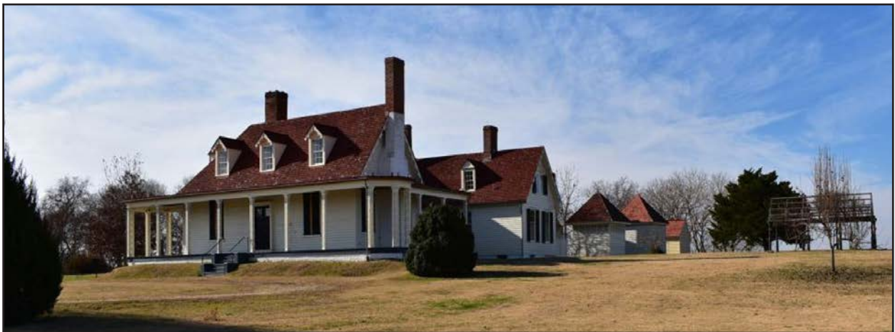
Figure 67. Appomattox Manor (116-0001), main house and outbuildings, looking west, 2018 (V-CRIS).
