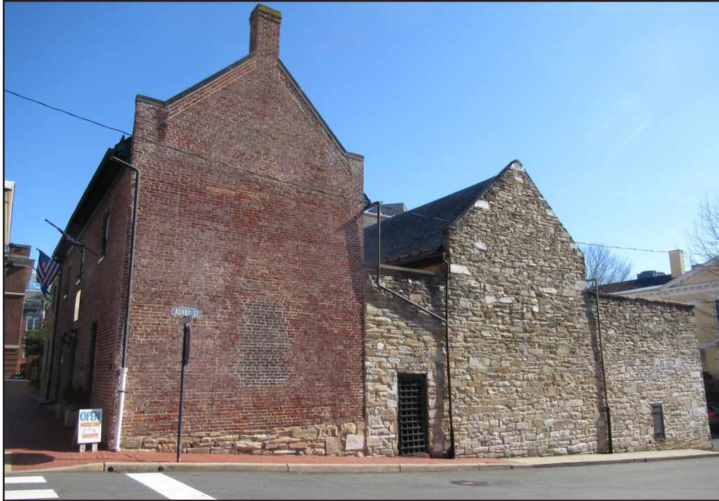
Figure 58. Fauquier County Jail (156-0004), northwest elevation.
