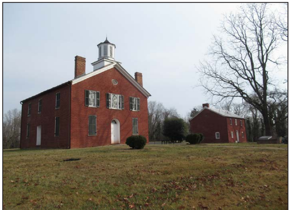
Figure 96. Brentsville Courthouse complex (076 0021), with the courthouse on left and the jail on right, looking northeast.
