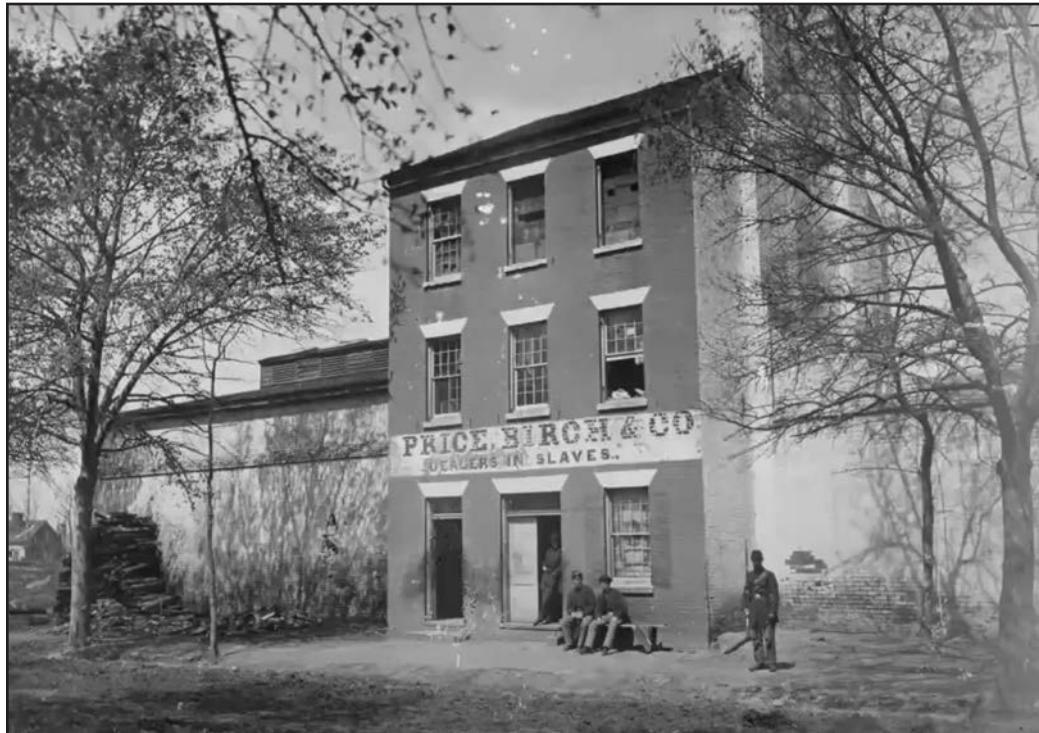
Figure 5. The offices and adjacent “slave pens” (holding areas) of dealers in Alexandria that specialized in the slave trade from Virginia to Natchez, Mississippi, and New Orleans, Louisiana.
