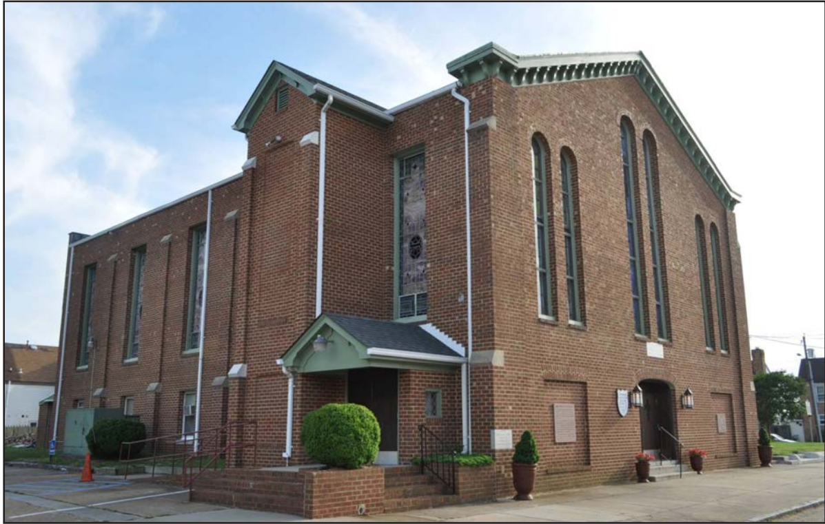
Figure 93. Emanuel AME Church) (124-0050/124-0034-0052), north and east elevations (Emanuel AME Church 2022).
