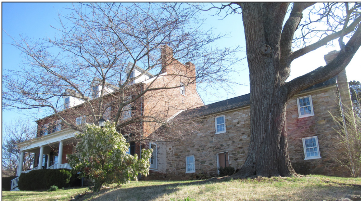
Figure 80. Melrose (053-0454), southwest corner of house.
