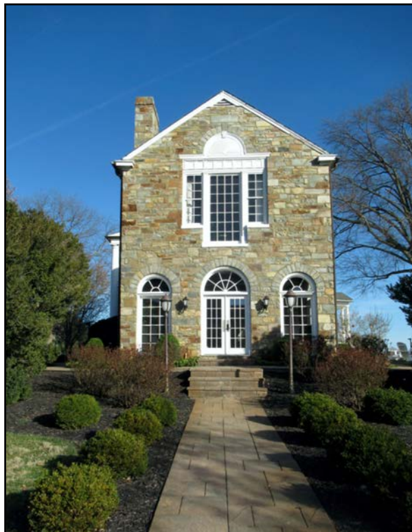
Figure 102. Evergreen (076-0007), west elevation.
