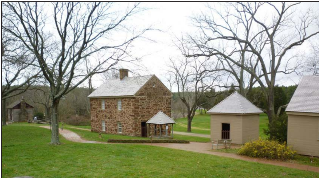
Figure 55. Sully Historic Site (029-0037), outbuildings (left to right: log schoolhouse [moved from Prince William County], dairy, smokehouse, kitchen).
