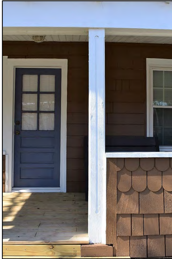
Figure 5. Porch support at 2517 Fentress Avenue (VDHR #134-5473/134-5672-0005) detailed with chamfered corners and an incised vertical channel with rounded ends.
