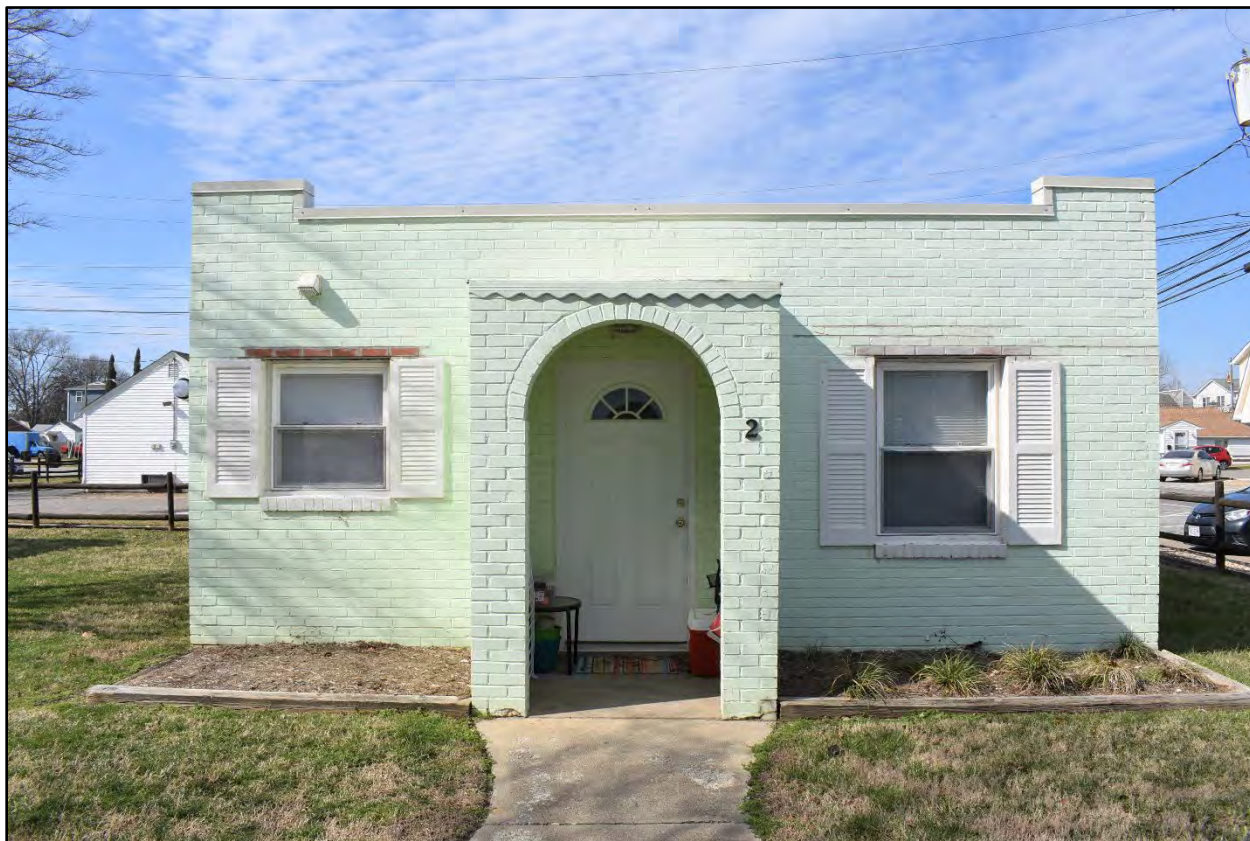
Figure 7. Looking West at Unit 2, Cottage Court, 4498 Lookout Road (VDHR #134-5479/134-5672-0010).
