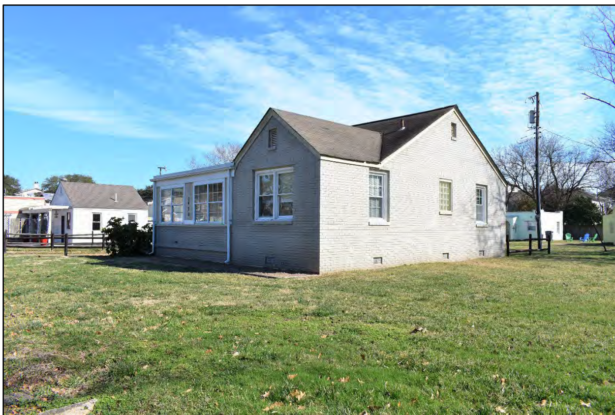
Figure 6. Minimal Traditional form house at 2420 Seaview Avenue (VDHR #134-5672-0036).
