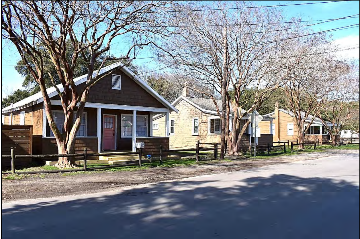
Figure 4. Row of three vernacular dwellings, or “beach cottages,” on the west side of Fentress Avenue.
