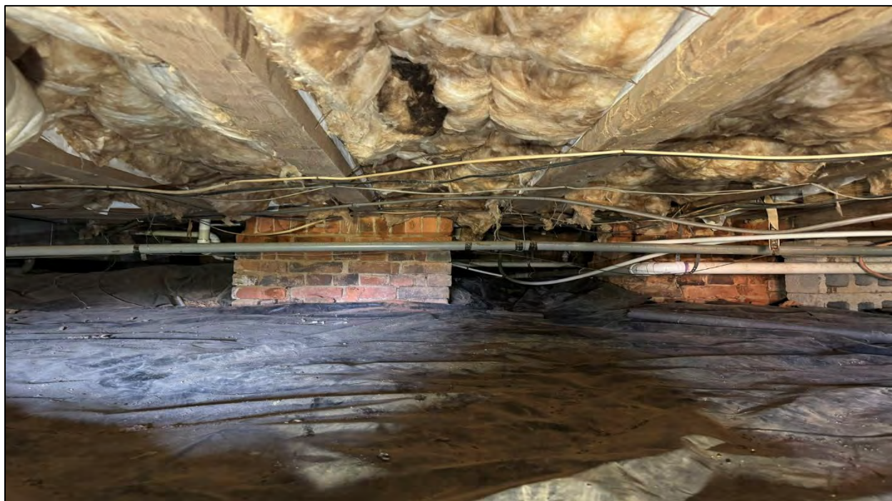
Crawlspace beneath the two-story section, looking towards the rear of the house at brick piers supporting the rear sill. October 2024.
