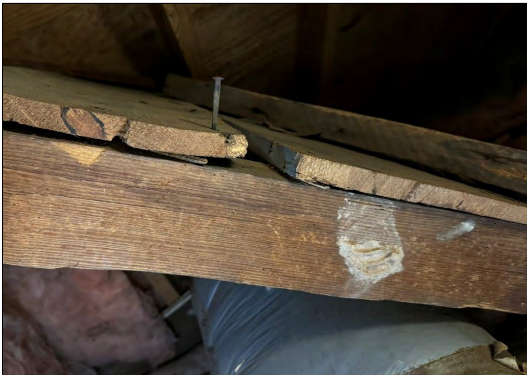
Rafter and original roof sheathing of the 1 ½-story hall-and-parlor section. With in-situ double-struck cut nail. October 2024.
