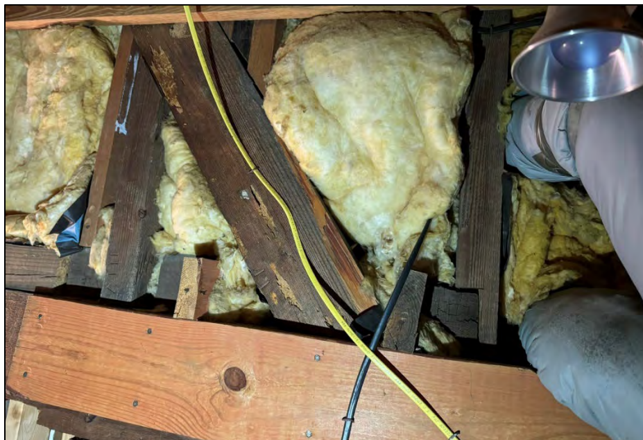
View of the framing associated with the original run of stairs. Same brace as is shown in the image above. Note the ends of the headers, one of which is notched into the base of a stud. Also note the carpenter's marks. October 2024.
