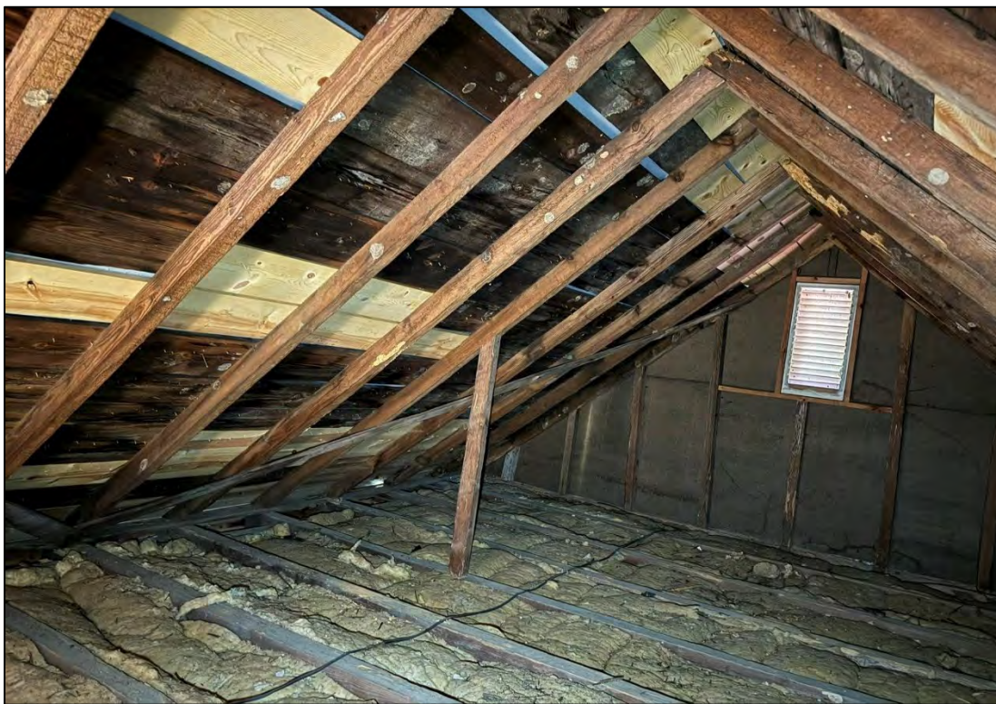
Attic of the two-story section. Looking at the west end wall. Showing diagonal bracing and rafters pegged at the ridge. October 2024.
