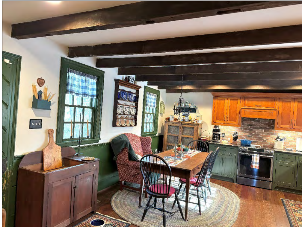
Kitchen, looking in from the hall doorway. Note the open mortises visible in the joist closest to the photographer marking the location of the former end wall of the kitchen ell. November 2024.
