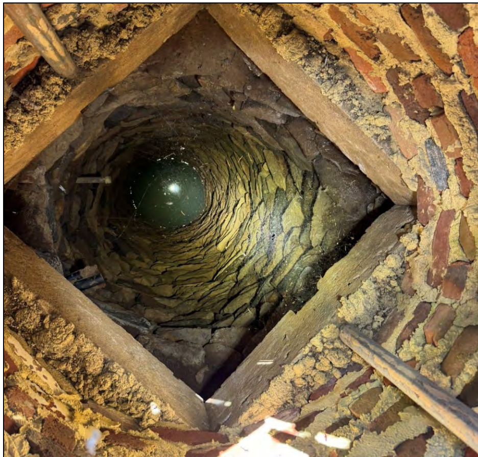
Looking down into the well at the 19 th century stone-lined portion. October 2024.
