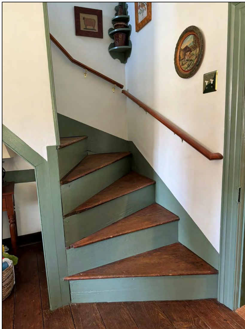
Stair in the hall-parlor section of the house. Notches on the left ends of the risers mark the former location of some type of newel or railing. October 2024.
