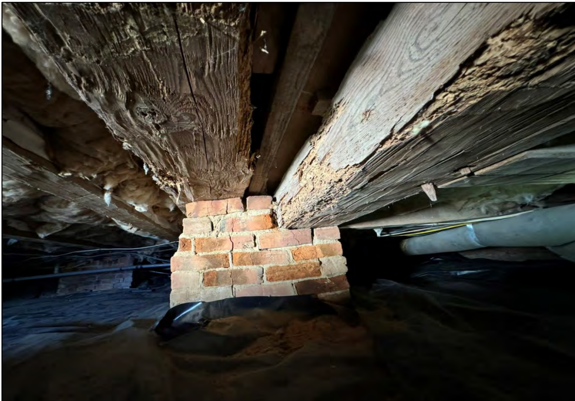
Crawlspace beneath the house. Brick pier supporting the sills of both the two-story section (on the left) and the hyphen (on the right). Note the pegged joint right of center that is the opposite end of the beam resting on the pier beside the chimney shown on a previous page. October 2024.
