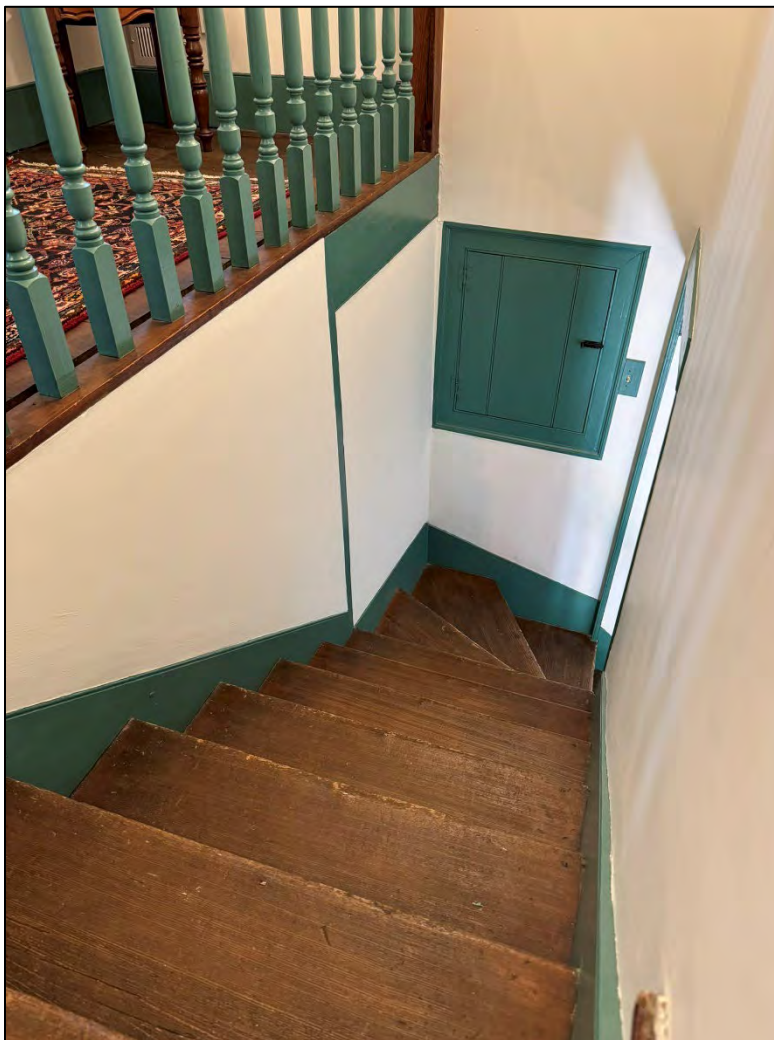
Stair in the two-story section of the house, looking down at the original header marking where the stairs rose from the opposite direction than they do now. Small door is the access to the attic above the lean-to. October 2024.
