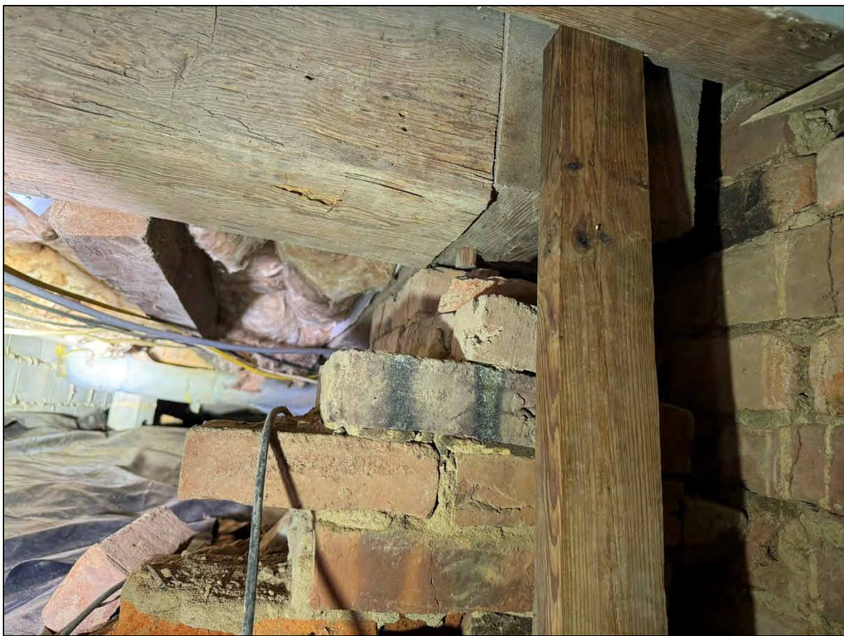
Partially collapsed brick pier, on the left, beside the chimney, on the right, showing the pegged joint of the two heavy beams that were supported by the pier. October 2024.
