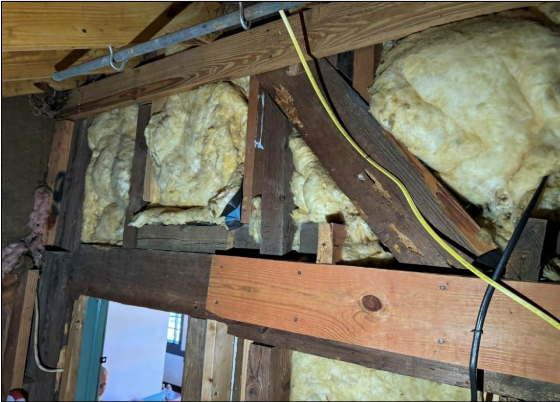
View of the framing of the back wall of the two-story section visible from the attic of the reconstructed lean-to. The dark-colored horizontal framing member in the middle of the photo is the girder supporting the second floor. Note the large peg where it intersects the corner post on the left of the photo. Also note the carpenter's marks on the diagonal brace and one of the studs. October 2024.
