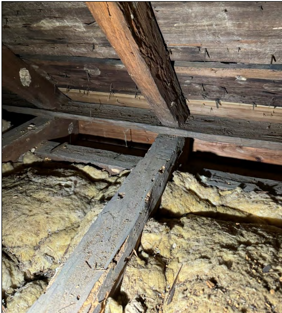
Attic of the two-story section. Common rafters sitting on a board false plate. Note the carpenters mark at the end of the joist. October 2024.
