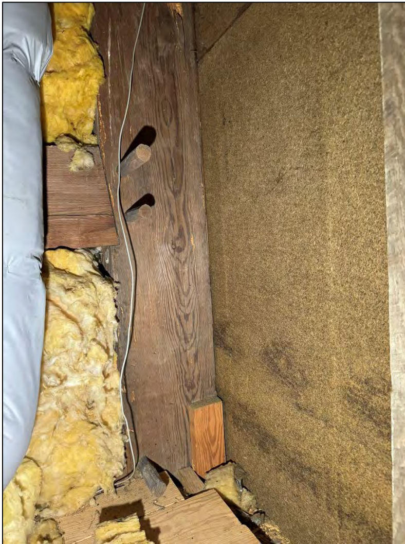
View of the framing of the back wall of the two-story section from inside the attic of the lean-to. Vertical beam is the northwest corner post, horizontal beam pegged to it is the girder supporting the second floor. October 2024.
