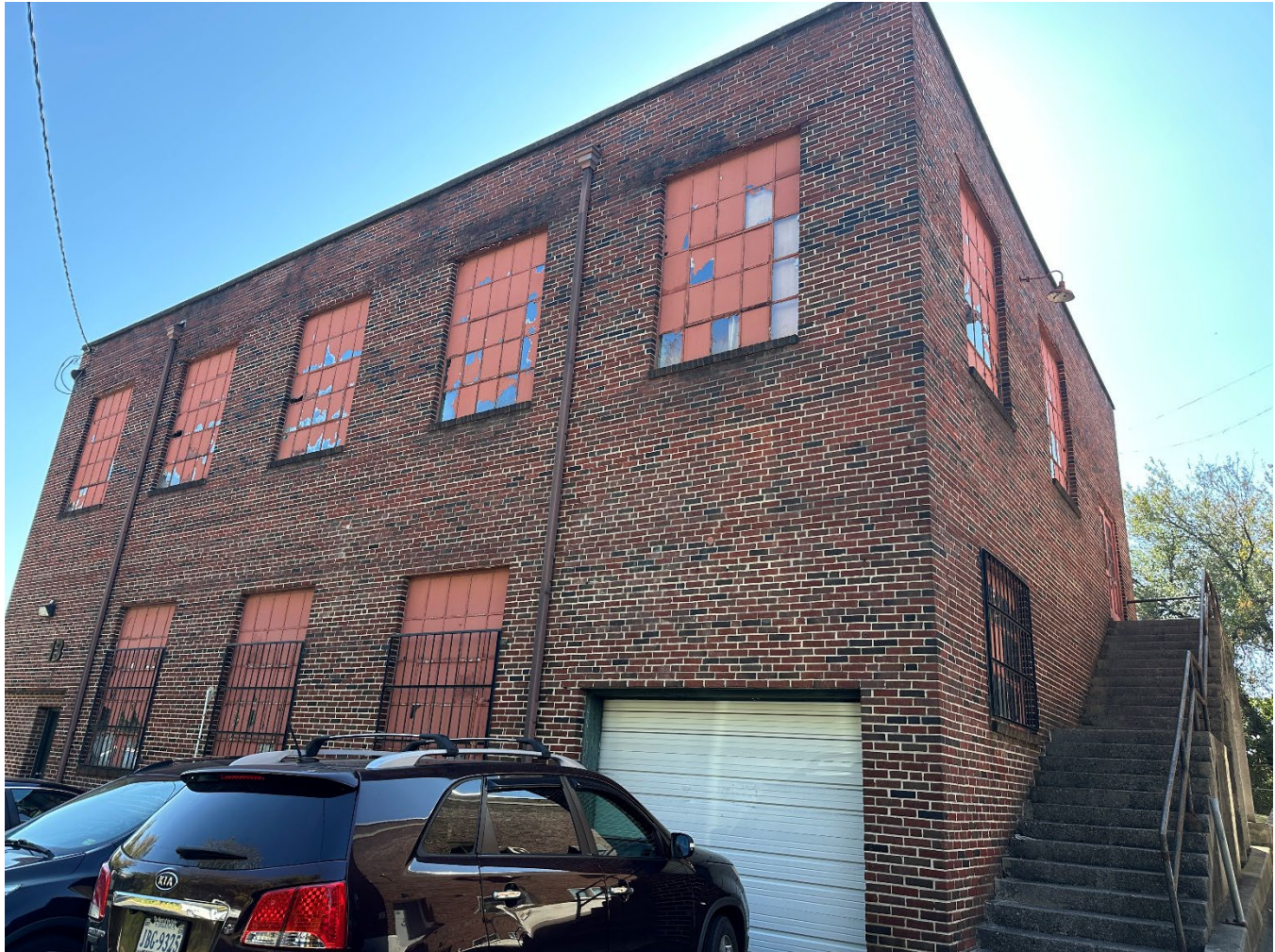
Figure 6: Front entrance view of the industrial arts annex building prior to demolition, view southeast, October 2024.
