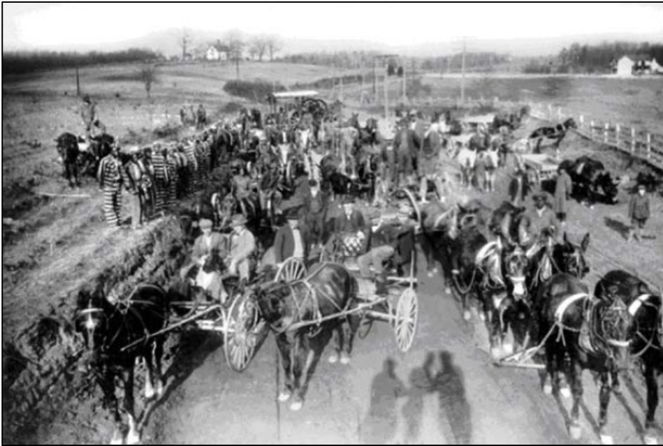
Figure 14. 1910s view of a road-building crew in Virginia that included convict labor, hired hands, supervisors, and mule teams; the horses in the foreground were for transportation, not draft work (Image Source: Ann B. Miller and John E. Wells, "Baksights:" Essays in Virginia Transportation History, Vol. 2 (Richmond: Virginia Department of Transportation, 2011), p. 52.
